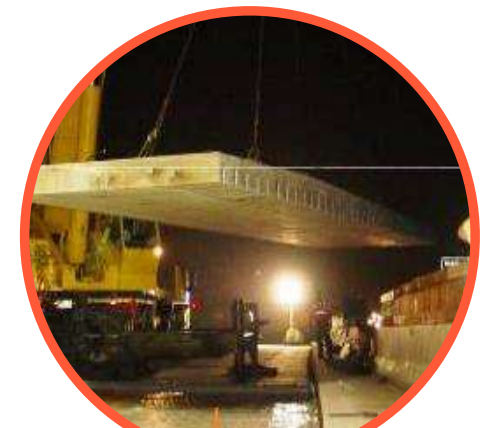
Replace distressed pavement with precast slabs
