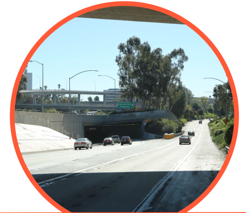
Resurface the pavement to create a smoother driving surface
