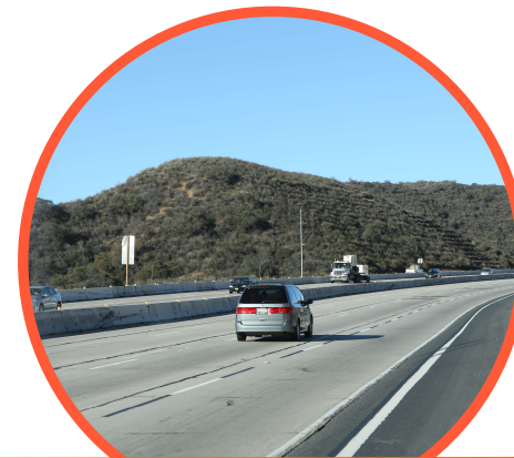
Upgrade the median concrete barriers and guardrails
