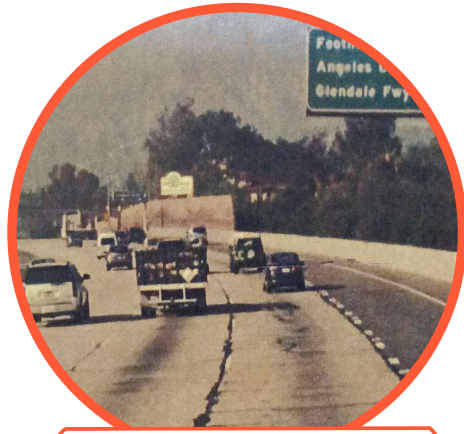
Upgrade signs and sign structures
